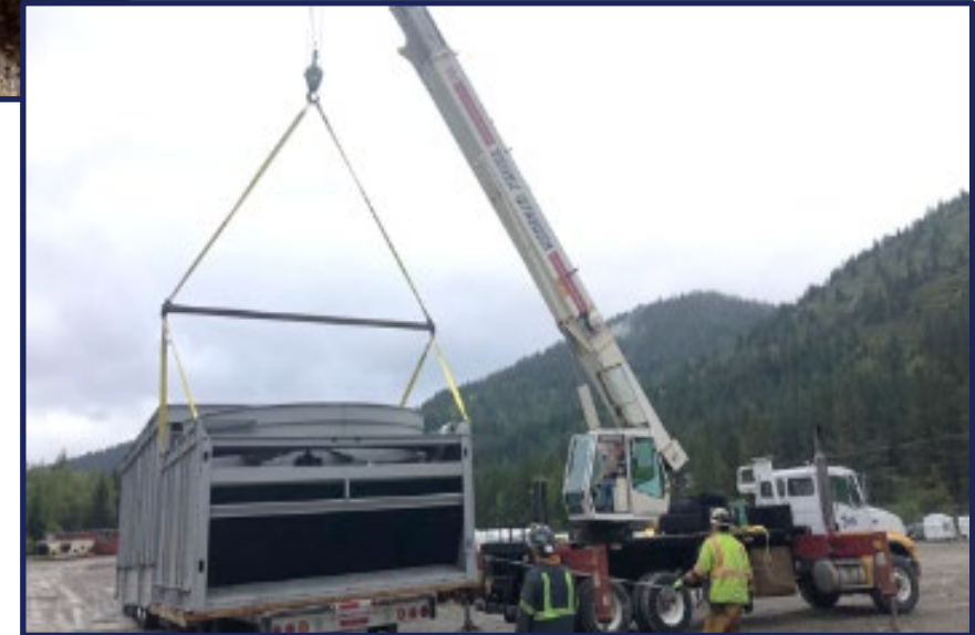
Surface Cooling Project
