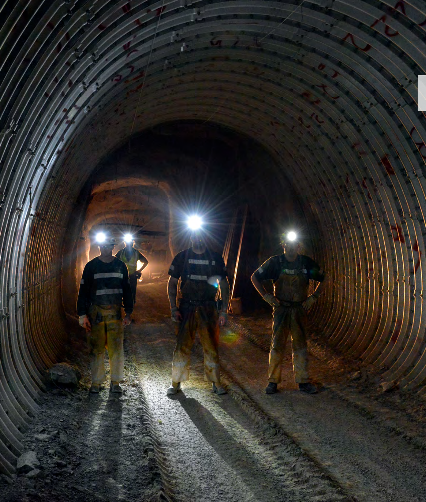
Workers in the newly built bypass drift on the 5900 level at the Lucky Friday silver mine in Mullan, Idaho.
